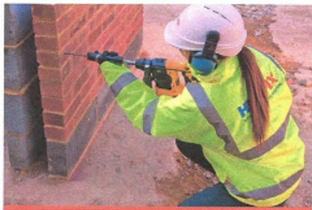
DryFix tie being power-driven into pilot hole
